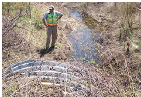
Exterior view of existing culvert
