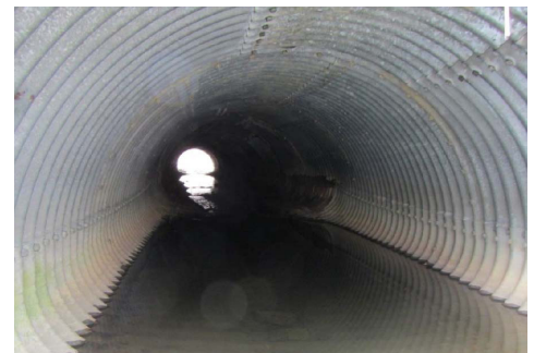
Interior of existing culvert 64-1N
