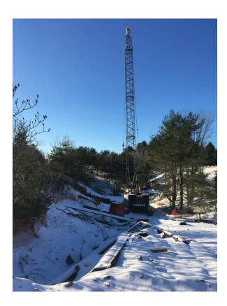
Crane preparing to lift steel framework for a cofferdam (known in the tunneling world as a Portal) located in the median between northbound and southbound I-89 travel lanes.
