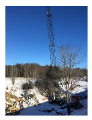
Crane used to install the steel sheeting and framework. When this portal is complete, the crane will be moved to the northern end of the project to install the second of three portals.
