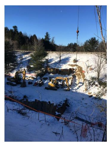
Median cofferdam sheets exposed. The area within the steel sheets will provide a contained area for tunneling operations starting in the spring of 2017.
