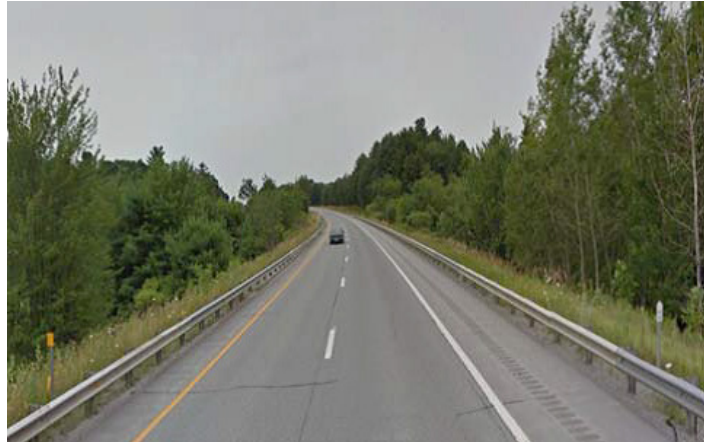
View of I-89 over southbound culvert
