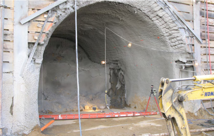
Example of trenchless construction
